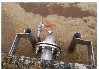
In case single aeration grids will be installed the purge can be connected either at the far end of the header or at the beginning at the lower end of the drop pie, both options will have the same function.
